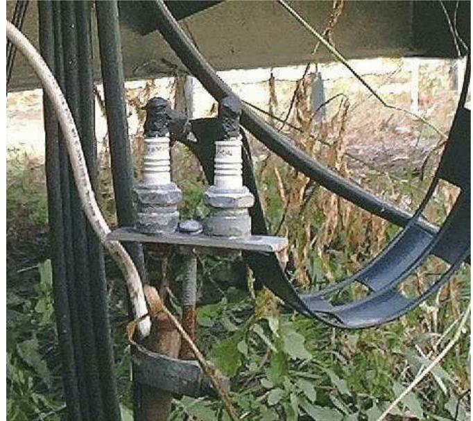
Figure 1 – Note the use of spark plugs as lightning protection
