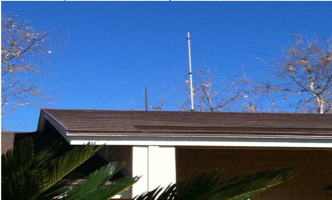
VHF/UHF vertical and HF "inverted-v" dipole as seen from the front yard
