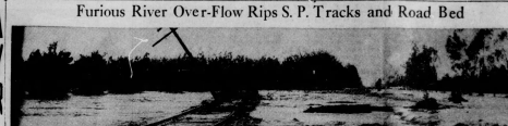
Furious River Over-Flow Rips S. P. Tracks and Road Bed Flood waters that have not only swept bridges to wreckage and power lines to fall left Santa Ana and the towns isolated from the rest of the world. The water was so high that it was over the hills and across the ridges.
