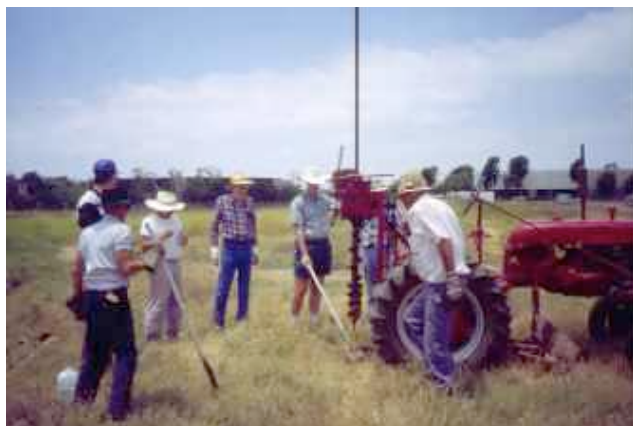
Kei-W6NGO in the white shirt on the right would bring his tractor (1996 is shown here) to dig tower base-holes at FD. "How many supervisors are needed to dig a hole?"
