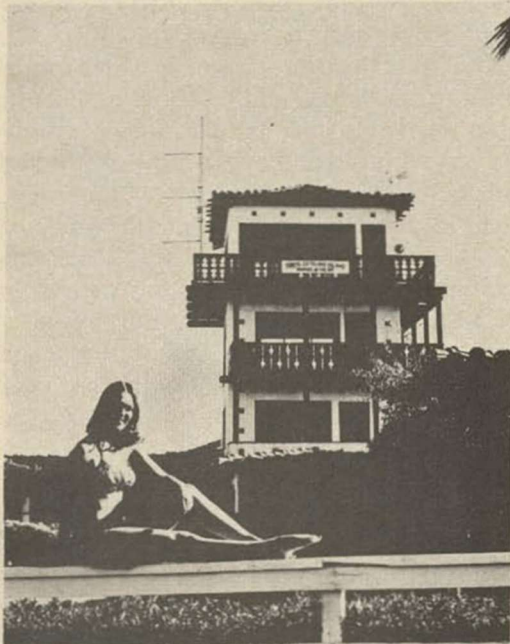
Catalina Airport Control Tower.
